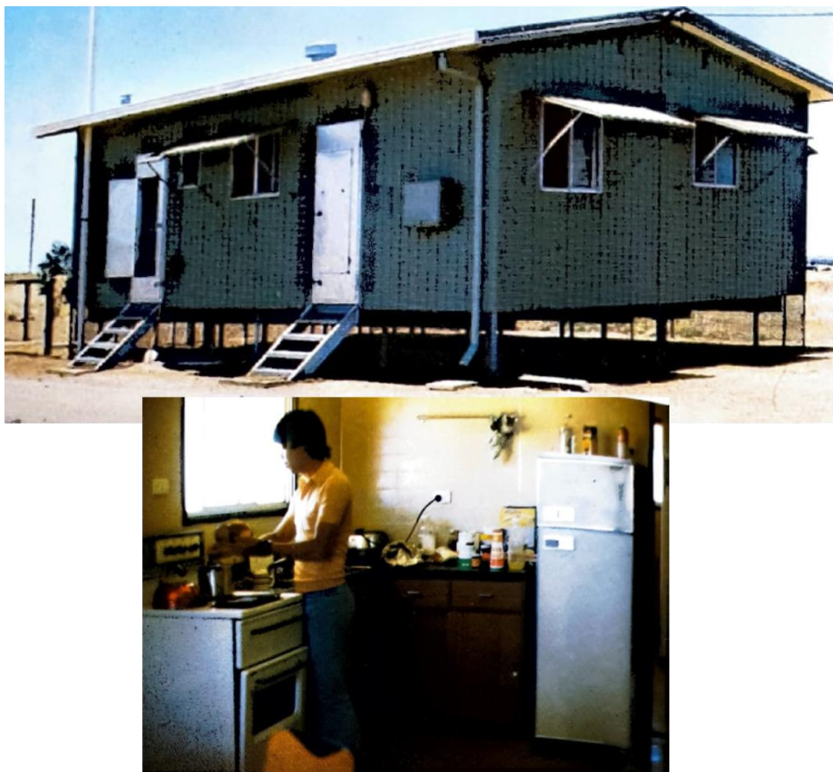
Figure 20: CBH receival point accommodation, 1975
