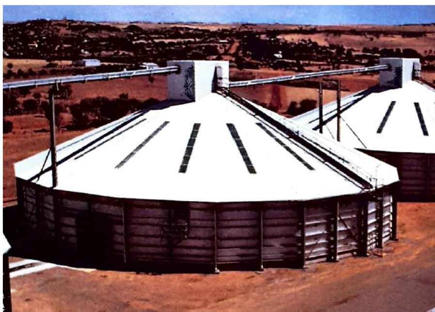
Figure 27: The “M Type” grain silos Northampton, 1990
