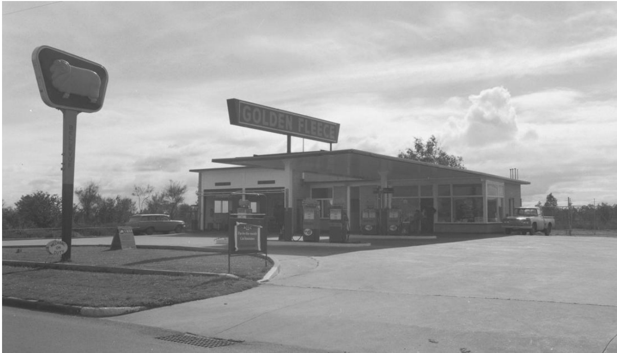
Figure 4: Golden Fleece Service Station, Bellevue, Western Australia
