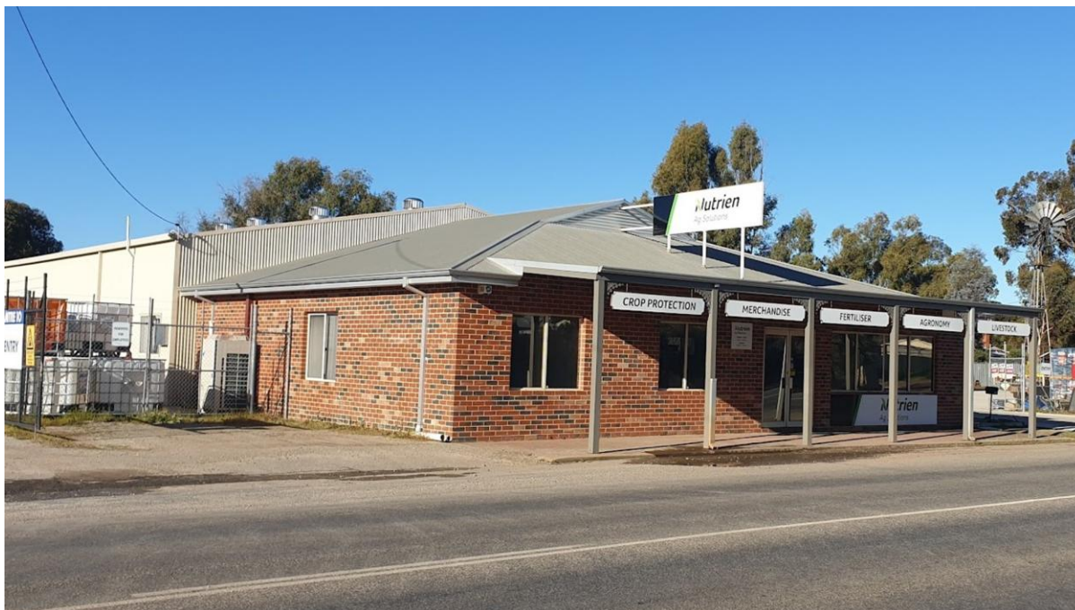
Figure 35: The York Rural Trading building 46 Avon Terrace
