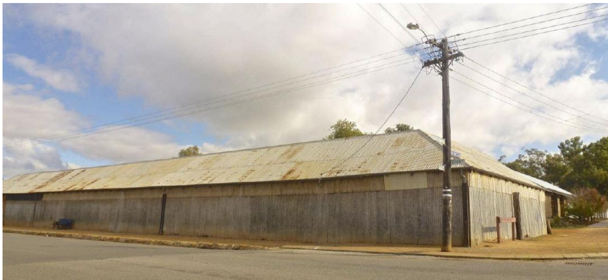
Figure 18: Monger’s Trading Post wagon yard and stables, 179 Avon Terrace York WA
