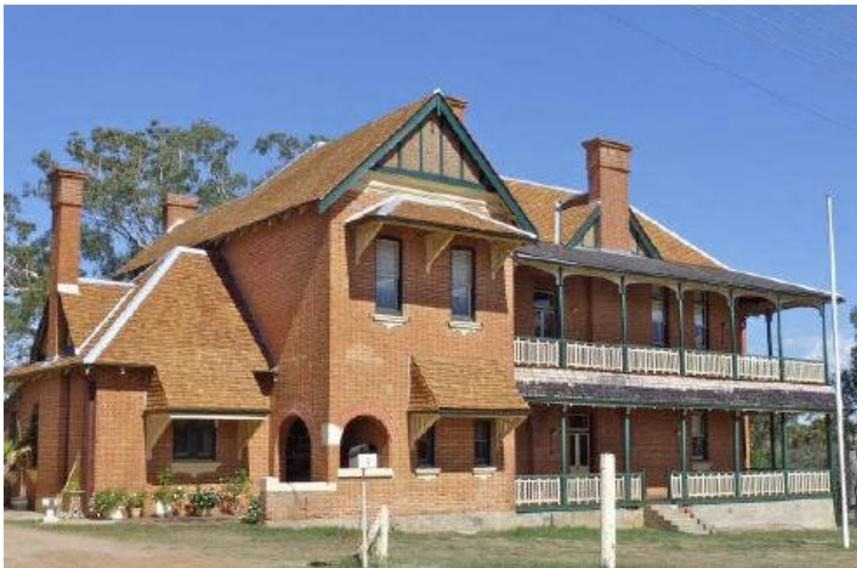
Figure 31: Old York Hospital
