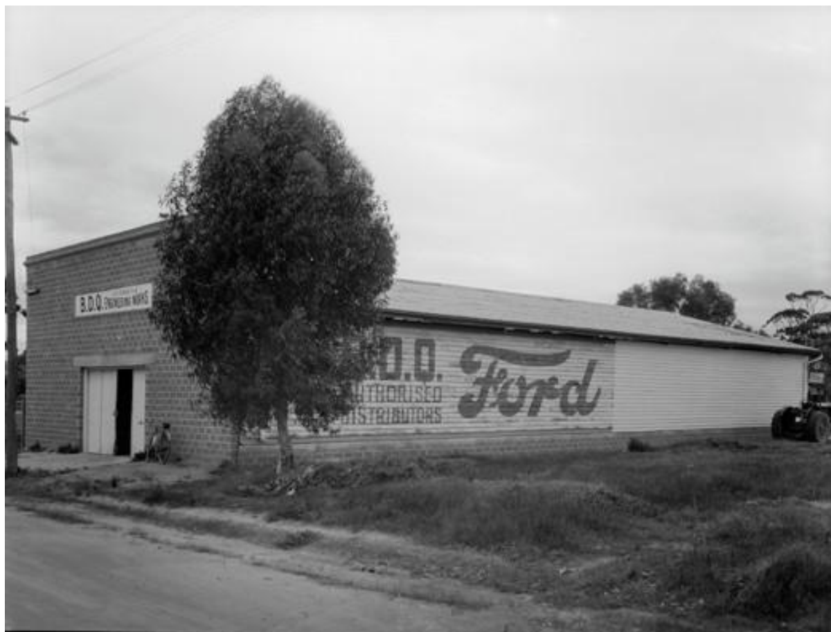
Figure 18: BDQ Engineering Work, Quairading 1953
